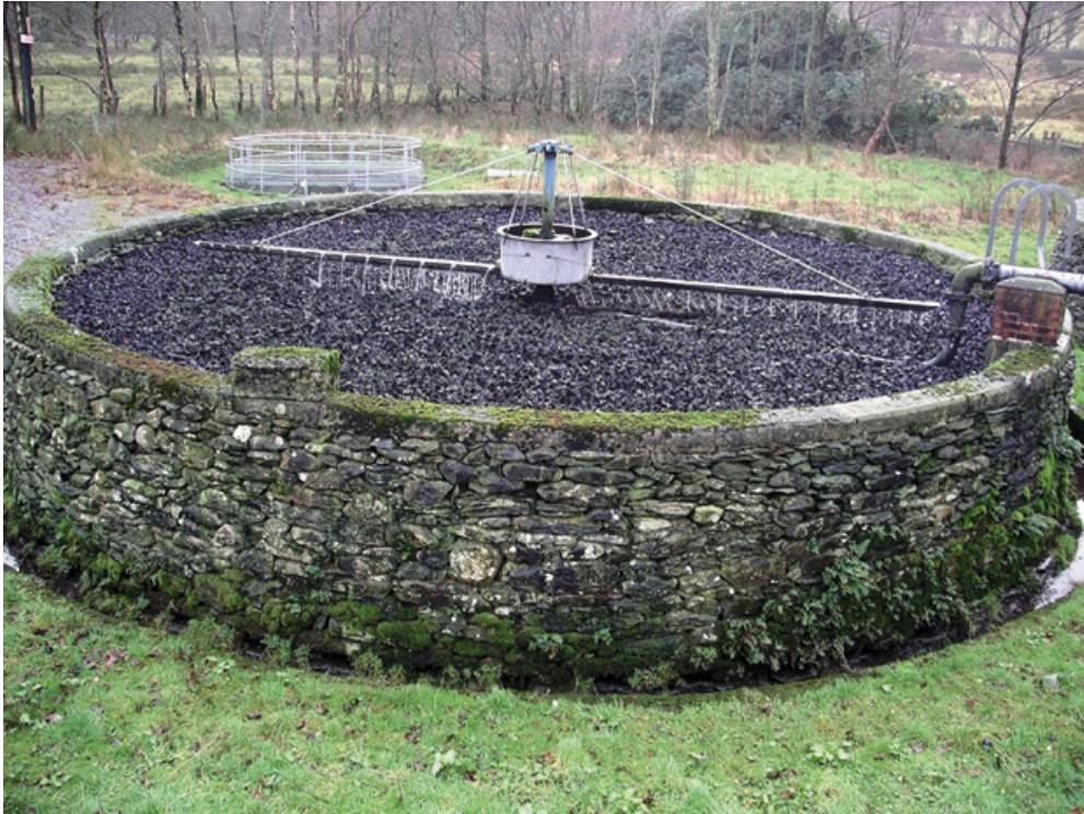
Plate 1.2. Biological trickling filter at rural STW
