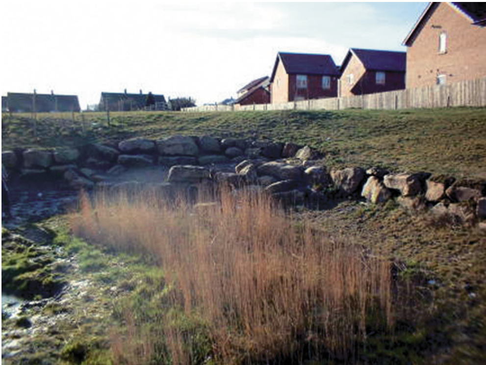
Plate 1.3. Typical reed bed treatment system (c)YES Reedbeds 2007
