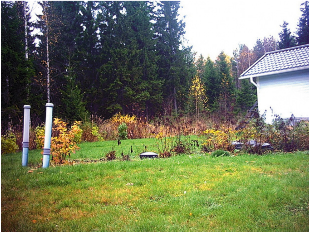
Figure 6. A buried sand filter. Photo Arja Ruokojärvi.
