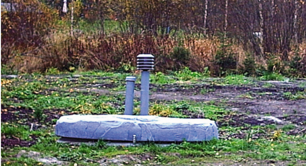
Figure 7. A package plant. Photo Arja Ruokojärvi.
