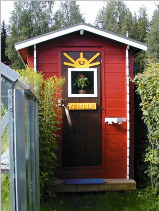
Figure 14. Dry toilets can be used in all properties. Photo Tuula-Anneli Kinnunen.
