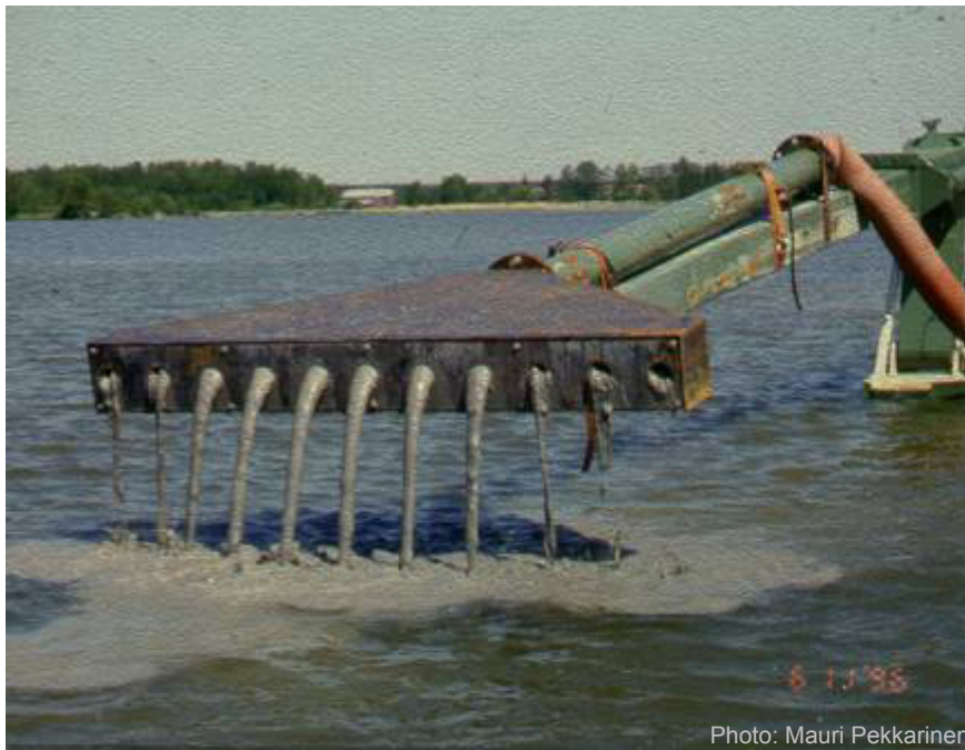
Figure 11. Nozzle for spreading clay
